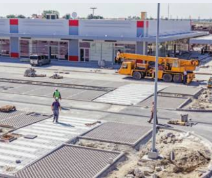
Building a new supermarket
